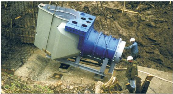
Instalace turbíny VC 1220 do MVE Kulišėnai (Litva) Installation of turbine VC 1220 into small hydro power plant Kulišėnai (Lithuania) Монтаж турбины VC 1220 - МГЭС Кульшенай (Литва)
