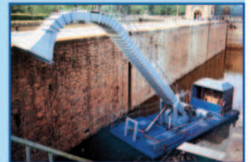
• Spillover small hydropower plant
