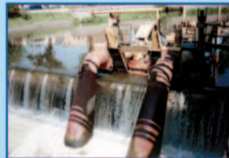
• Floating power plants with turbines Sigma 750 and Banki 600/1200
